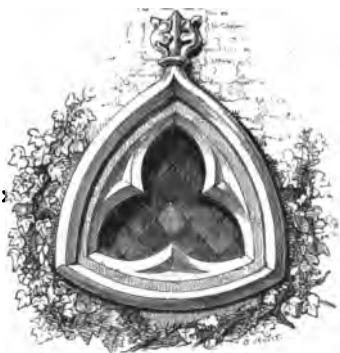
121. Cranford St. Andrew, Northants, c. 1320 Clear-story Window of the form called a spherical triangle.
